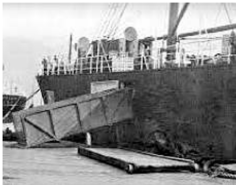
Loading ramp to Main Deck
